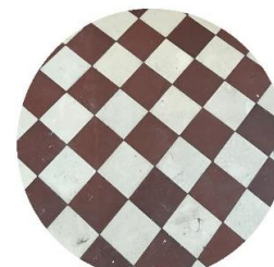
Carreaux de ciment 85m 2 2 tonnes
